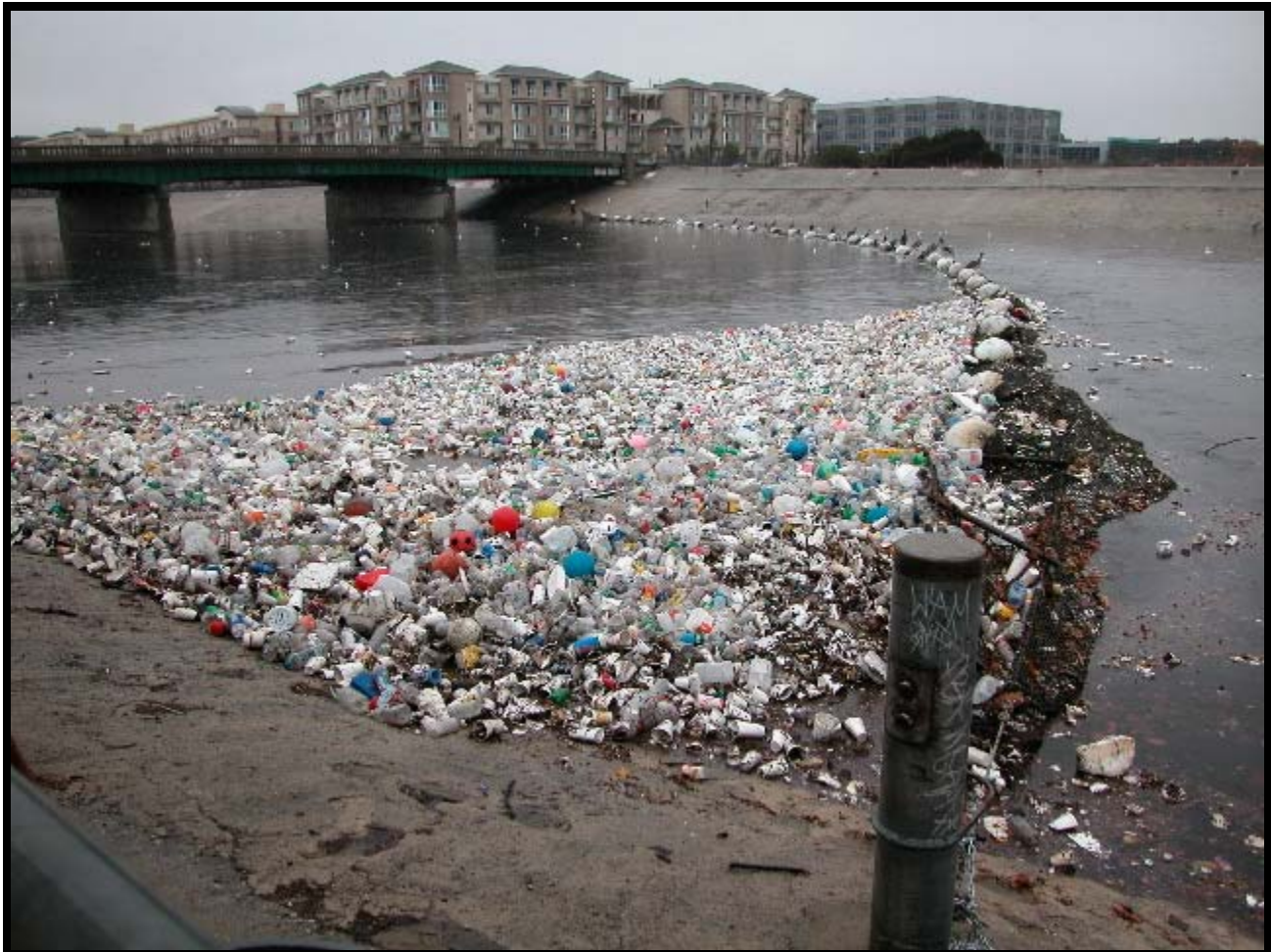
Trash net across typical Southern California Channel
